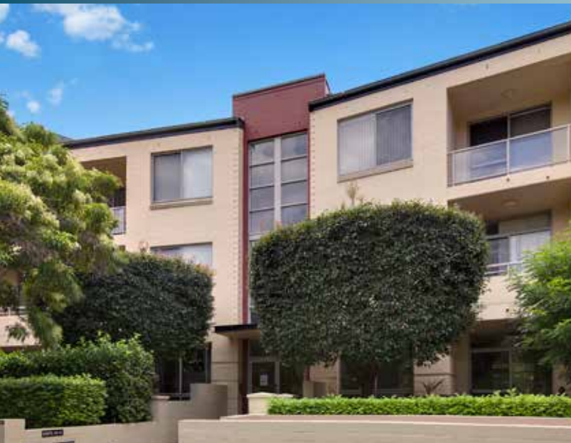
46/1 Kings Bay Avenue, Five Dock
